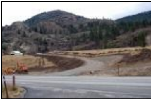
The new access road into the Whistler Canyon Trailhead. Its Done!
