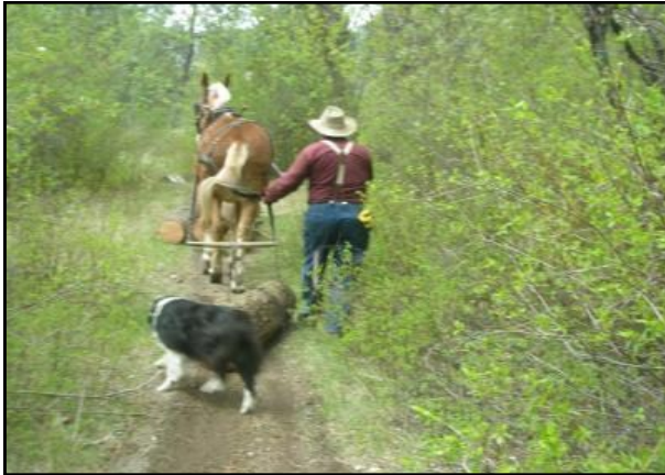
Stan Kvistad with help from Knute and Harley skidding stringer logs for the Whistler Canyon bridges
